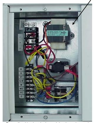
Fan coil unit's electrical panel that is exchanged with the kit's electrical panel
