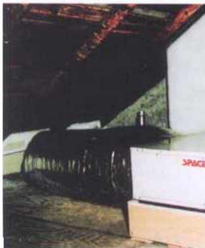
SpacePak's compact blower fits neatly into a small space such as attic, closet, or crawlspace. Inset: Flexible, insulated 2-in. dia. tubing disperses conditioned air from the blower to the rooms. The tubing is hidden between wall studs or ceiling joists like electrical wiring.
