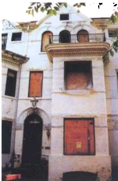
A fire gutted much of this Georgetown-area townhouse, which was later fitted with a SpacePak "high-velocity comfort" system.
