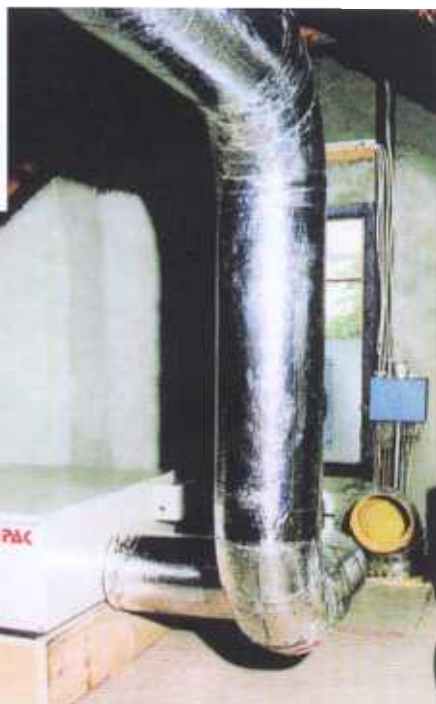
SpacePak's compact blower fits neatly into a small space such as attic, closet, or crawlspace. Inset: Flexible, insulated 2-in. dia. tubing disperses conditioned air from the blower to the rooms. The tubing is hidden between wall studs or ceiling joists like electrical wiring.
