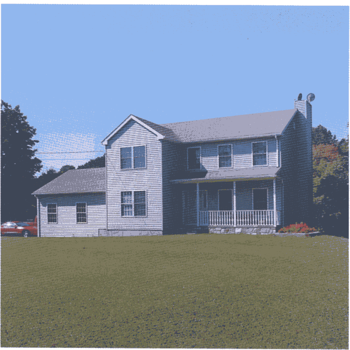
This home in Danbury, CT, uses the combination system, which is designed for maximum comfort and efficiency.
