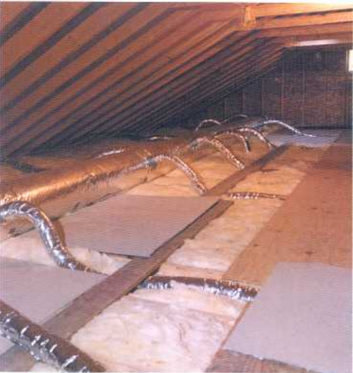
SpacePak plenum with 2-in.-id flexible ductwork delivers conditioned air to the living space.
