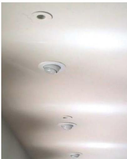
finished product are the small round air outlets – each about the diameter of a CD – which can be located on walls, ceilings or in floors. An air-handler unit is installed in the attic, basement or crawlspace. For this project, the air handlers were installed in the equipment room in the attached garage.
