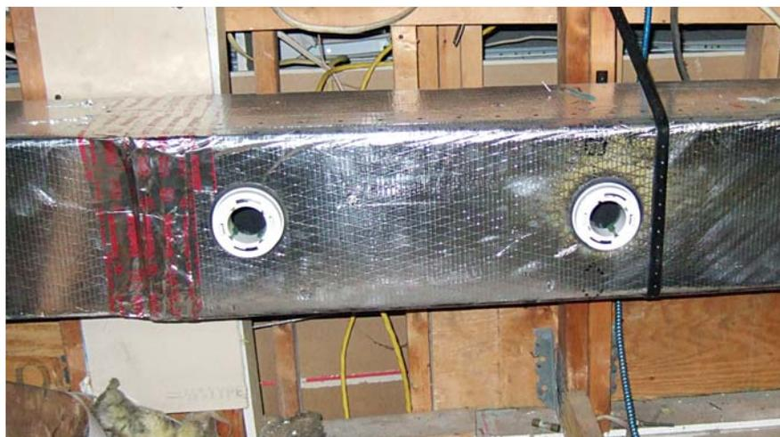
outlets can be installed through floors, walls or ceilings, and can be painted or covered with wallpaper. There are not any large ductwork systems that consume large amounts of space or the
